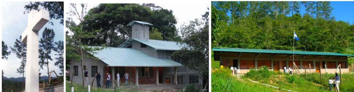
Figure 1: Reinforced concrete cross, volunteer center/chapel, the first classroom building.
